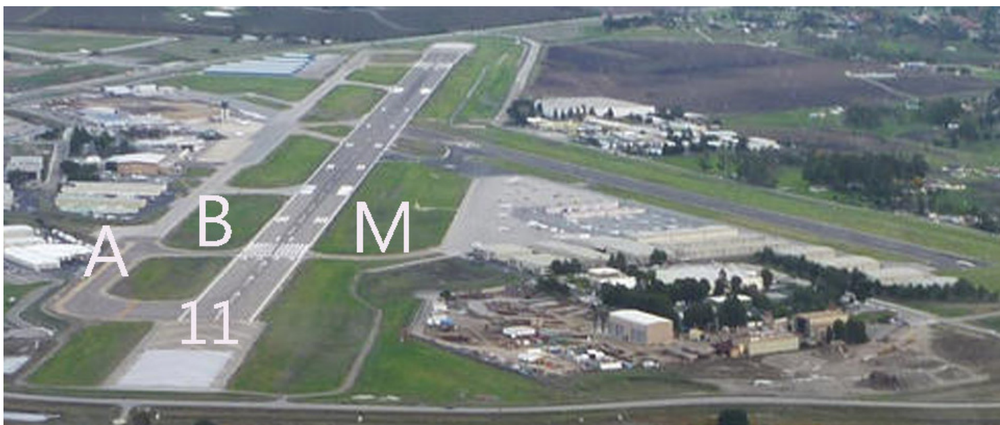
ILS critical area (see article on this page)
